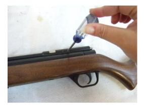
1. Remove the cam bolt plate from the R/S receiver
